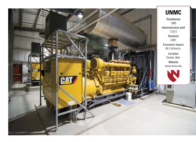
the operation of the generator sets and distribution circuit breakers. In the event of a power failure, a series of automatic transfer switches transfer the utility load to the generators, and maximum load is achieved within 10 seconds
